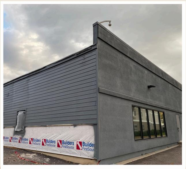
Project includes replacing the existing Masonite siding on the west exterior of SDSD with new siding and metal panel siding along the bottom. During the project it was preferred by SDSD to paint the entire building so it matched the west side.
